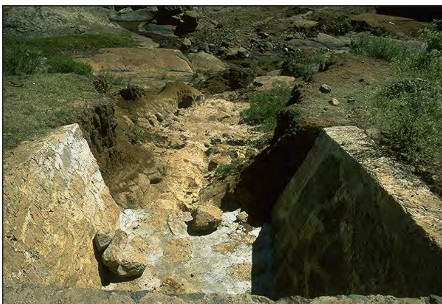
Photo 7.4 Add outlet protection and/or energy dissipators to prevent erosion and the formation of gullies.
